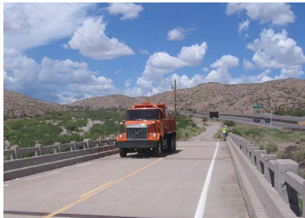
Fig. 8. A dump-truck used to excite the bridge.
