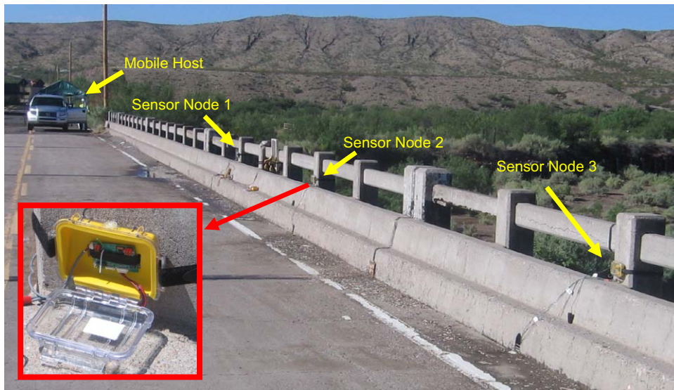
Fig. 9. Layout of the field test using WID2 conducted at the bridge.
